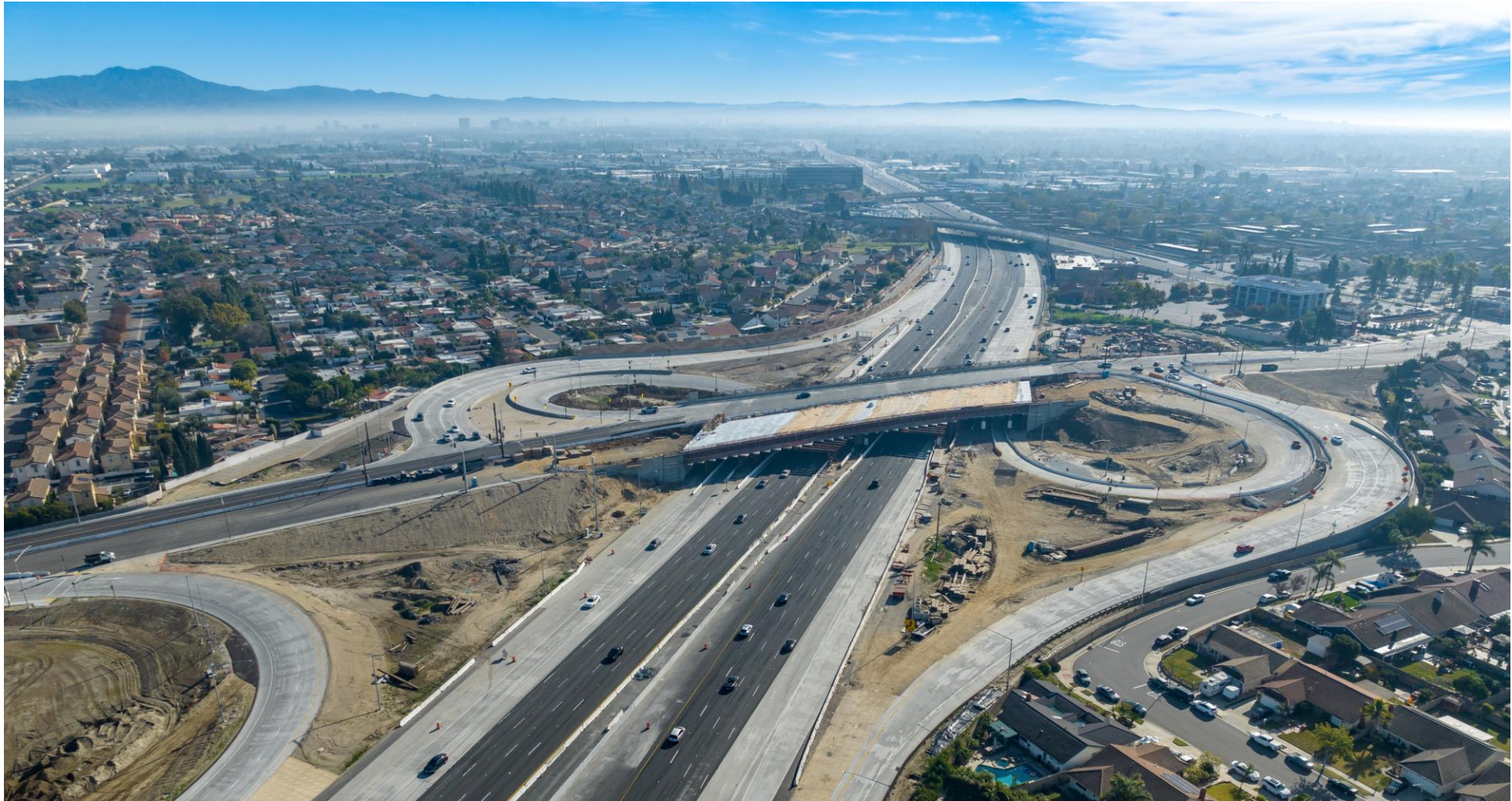
Brookhurst Street bridge construction
