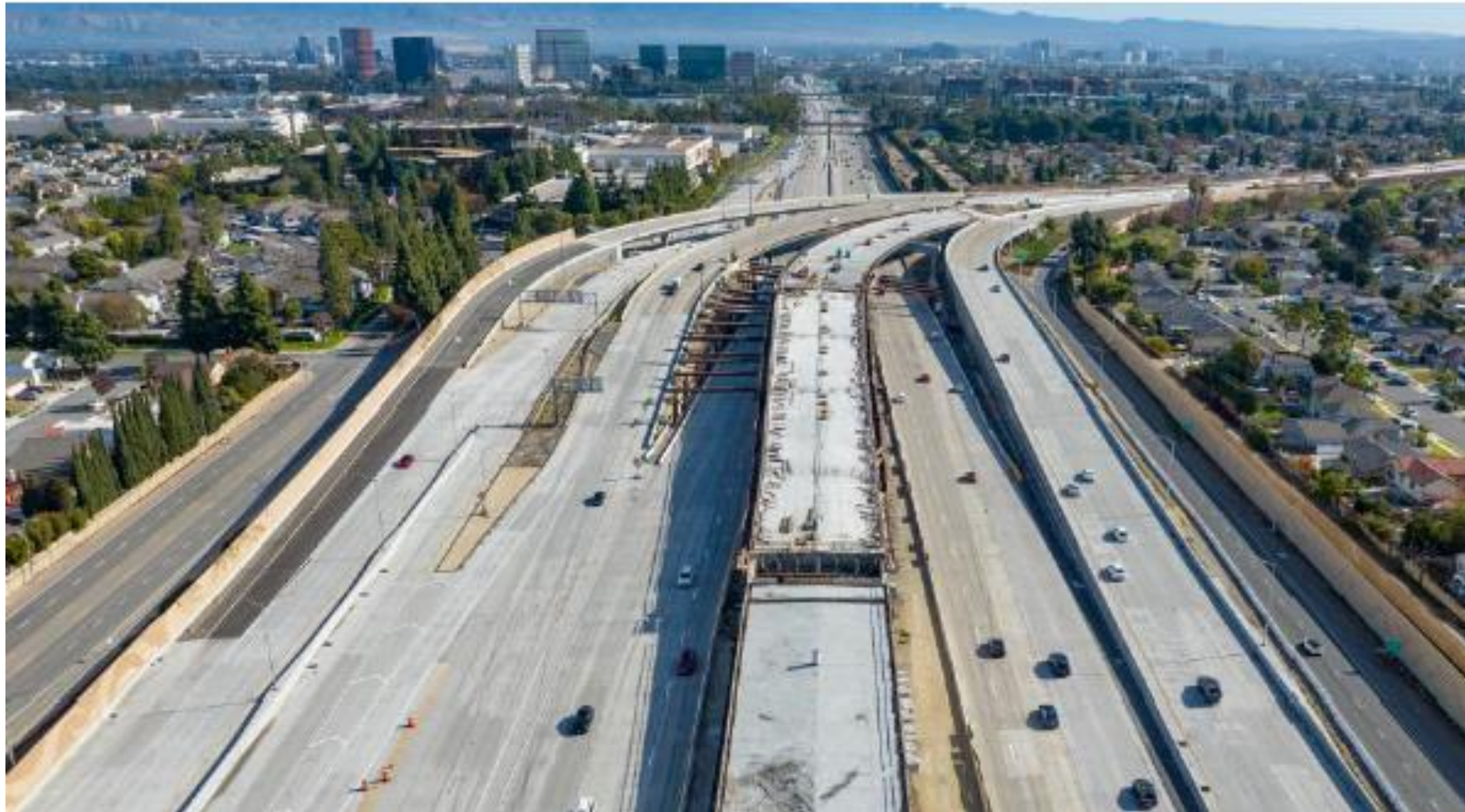
I-405/State Route 73 median connector bridge construction
