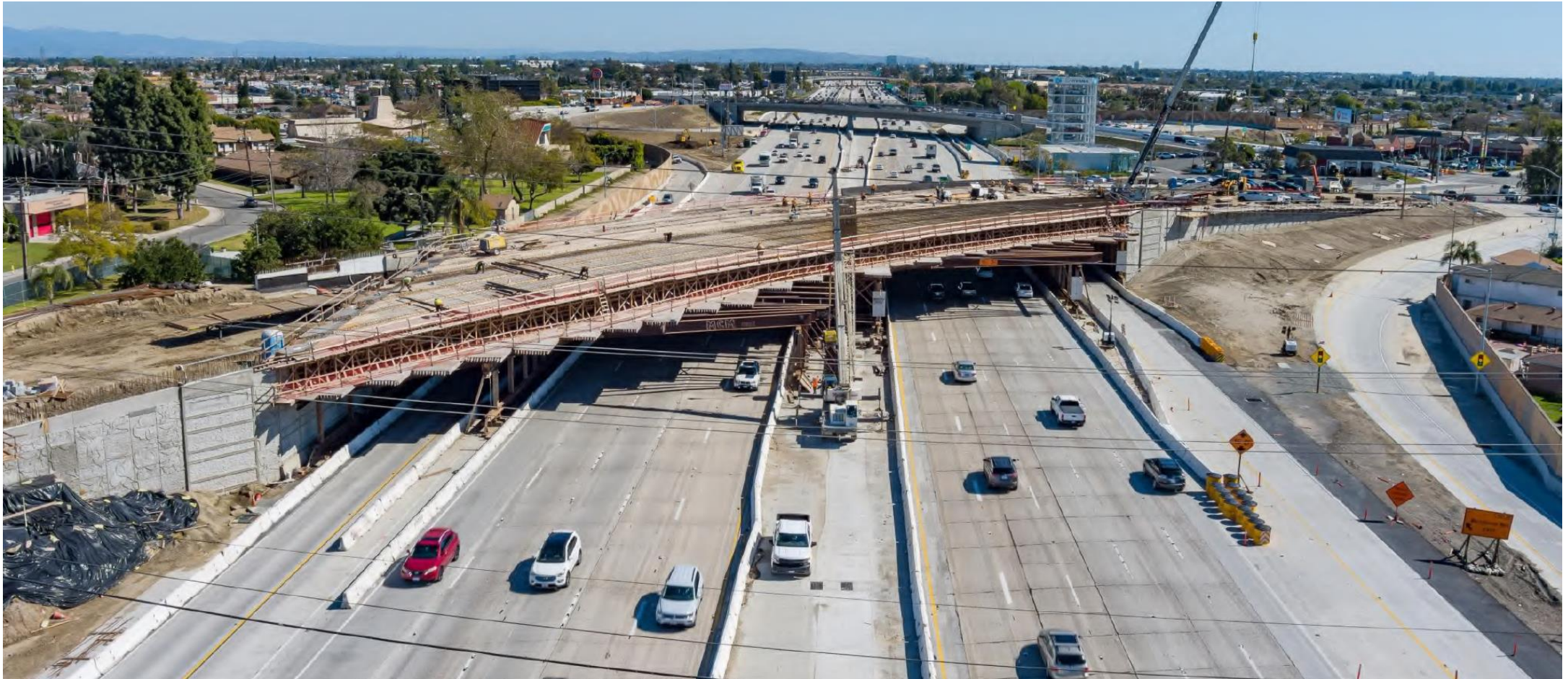
Springdale Street bridge construction
