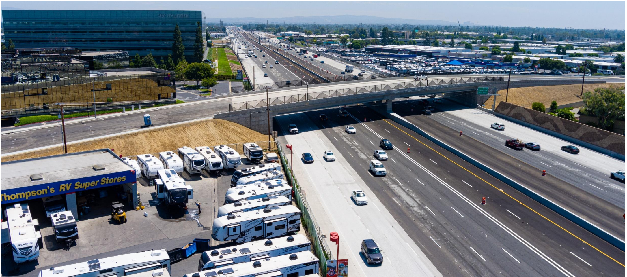
Ward Street bridge complete
