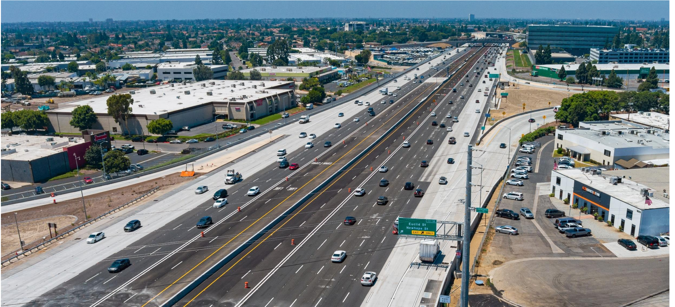
Express Lanes striping
