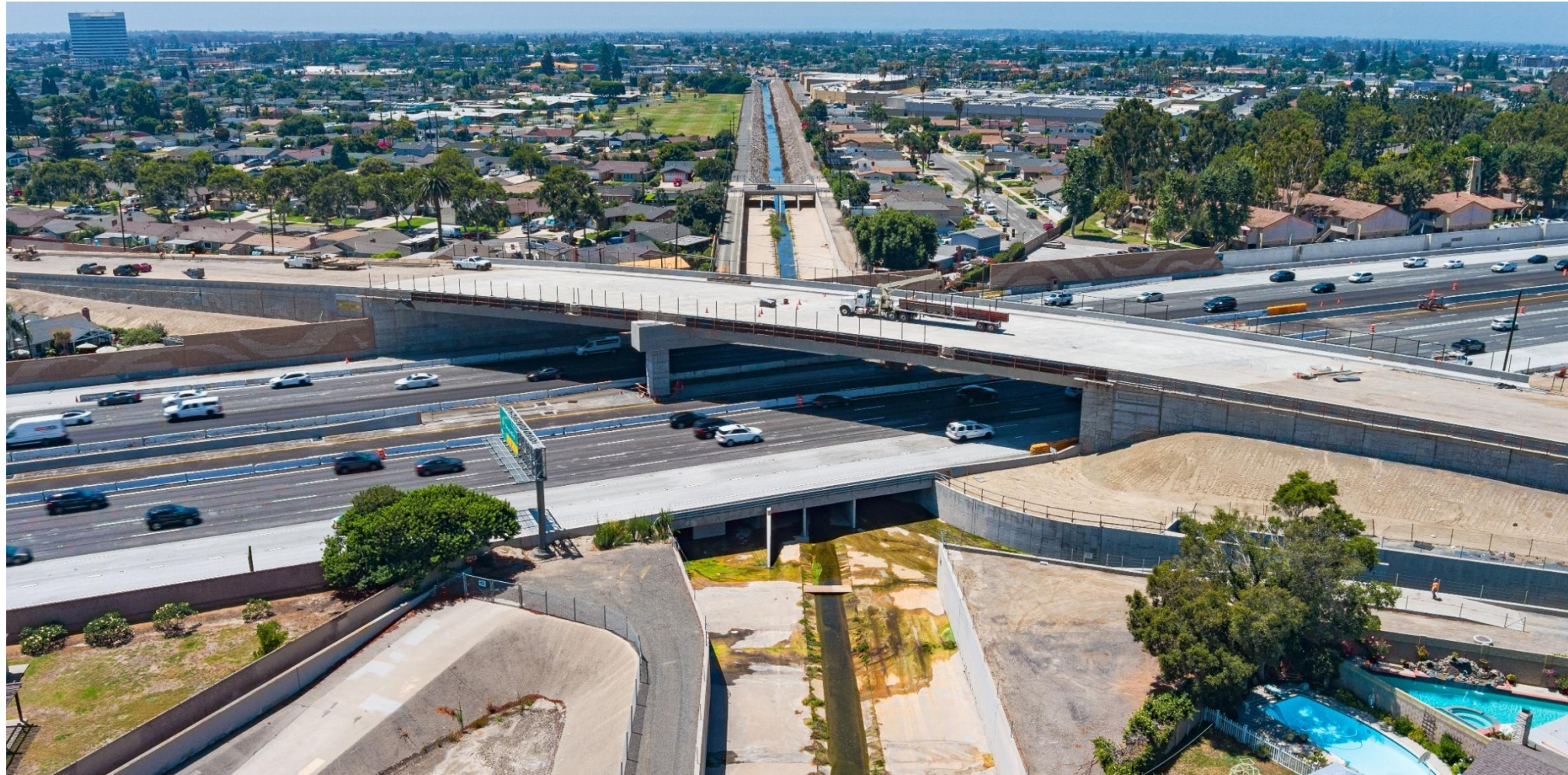
Newland Street bridge complete
