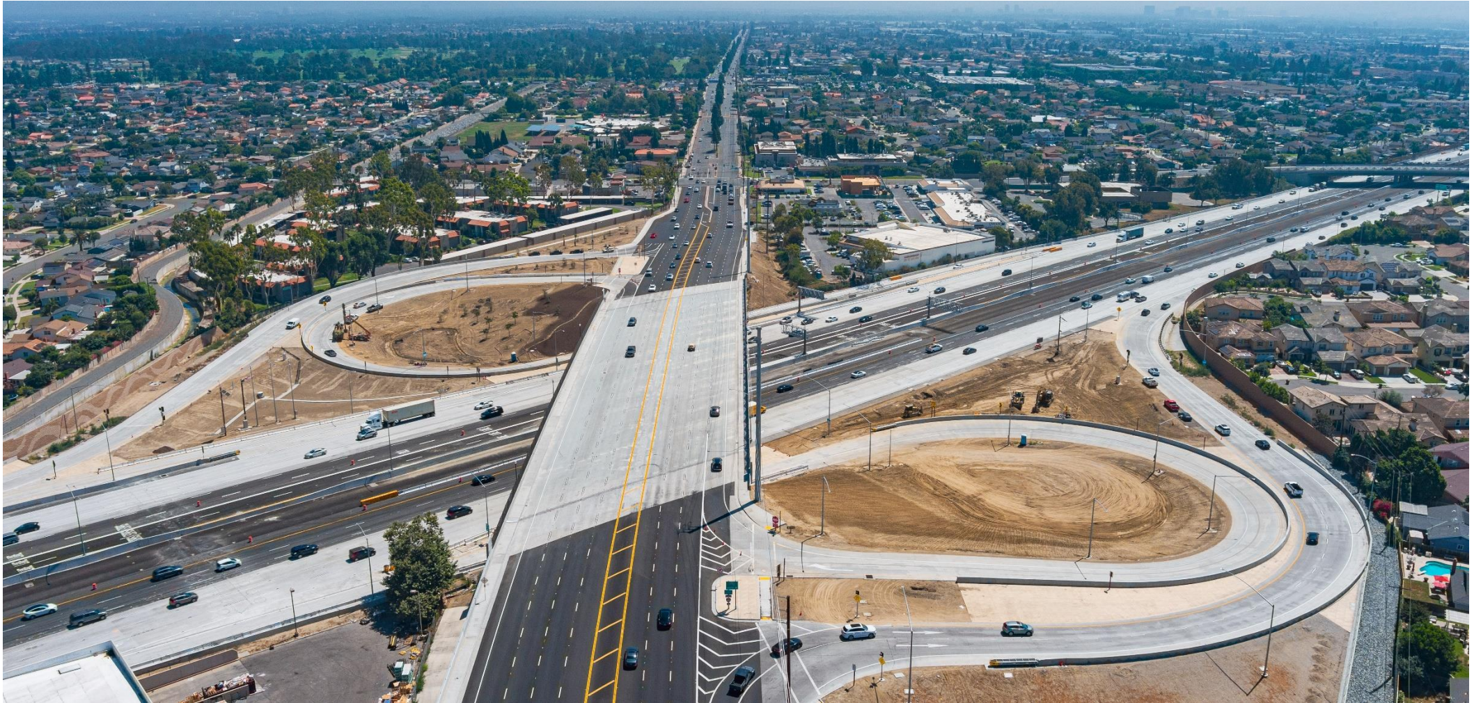
Warner Avenue bridge complete
